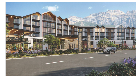
Hotel under construction
